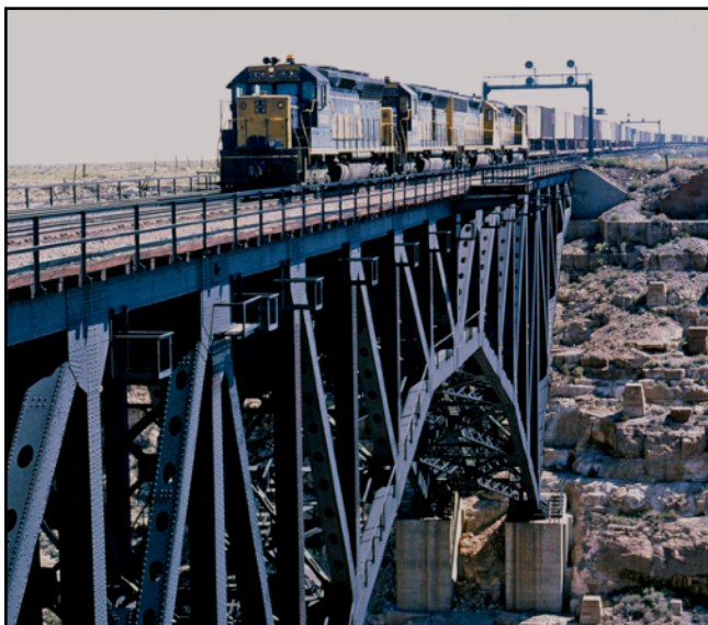
With strong winds kicking up desert sand, Santa Fe SD45 #5590 brings a hot westbound train across 1947-built bridge at Arizona's Canyon Diablo, October 1975. Old pilings of original 1881 bridge across canyon are visible on right. (Photo left)
