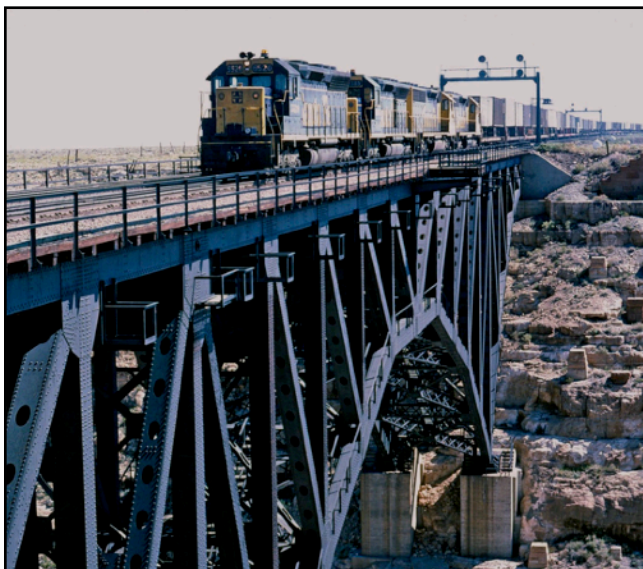
With strong winds kicking up desert sand, Santa Fe SD45 #5590 brings a hot westbound train across 1947-built bridge at Arizona's Canyon Diablo, October 1975. Old pilings of original 1881 bridge across canyon are visible on right. (Photo left)
