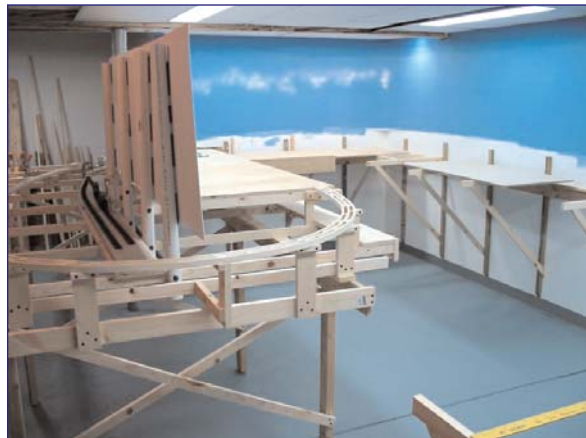
Center backdrop supported by PVC pipes
