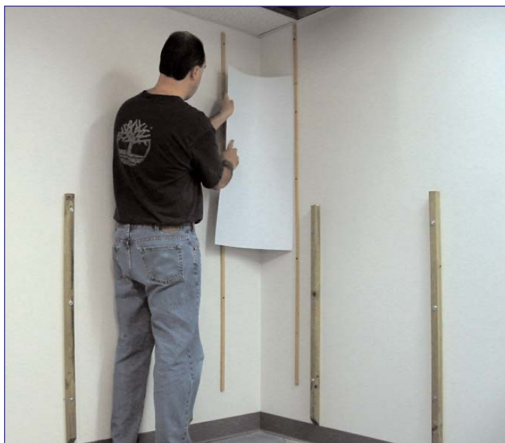
Curving the styrene into place
