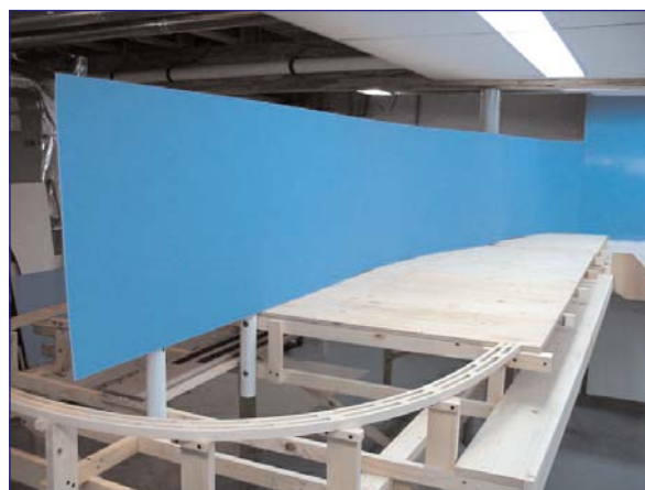
Center backdrop completed
