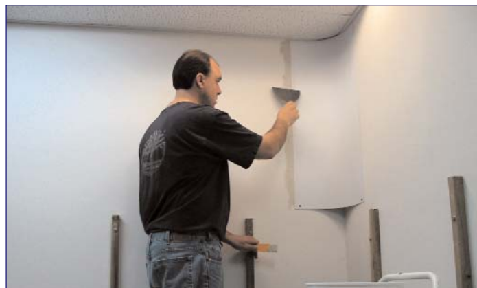
Applying drywall joint compound
