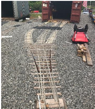
The tracks to the car maintenance area.
