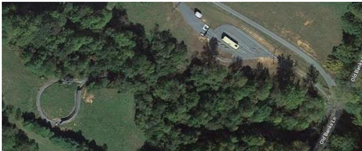
Aerial view of the BTIR
