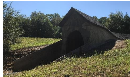
The 40-foot tunnel on the back loop.
