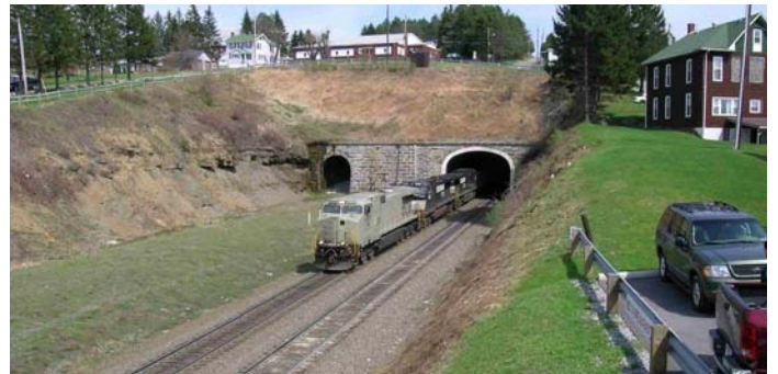
The Gallitzin Tunnels Photo by John Griffith
